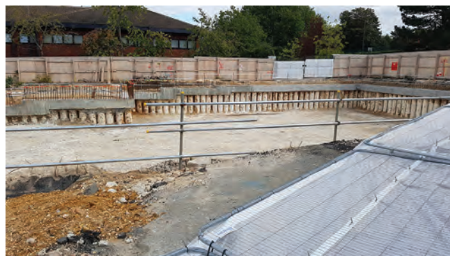
The basement after demolition of the building. Photo Howard Martin
